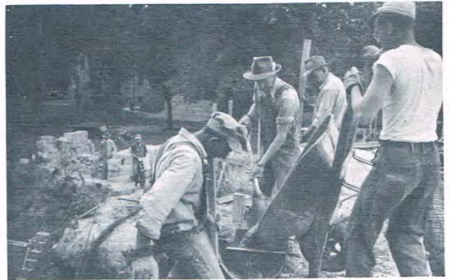
Pouring Foundation for Church Building
