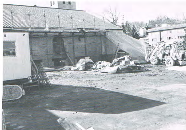
Construction site of new Narthex addition.
