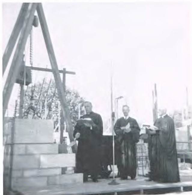
Rev. Eifert, Rev. Petzke, and Rev. Weinhold officiating at the Cornerstone laying of present church in August, 1949.
