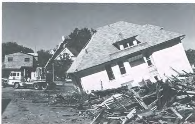
Demolition of houses for lower parking lot.
